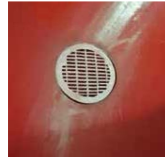
Waste water drain filter.
