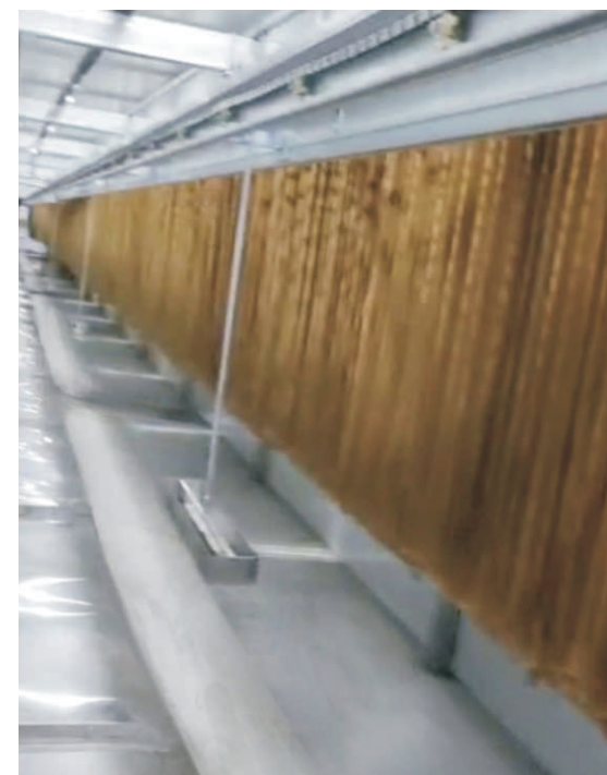
烘房 Drying Room
