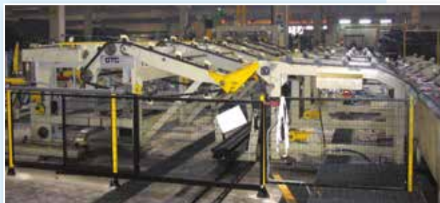
Impianto completo Complete plant
