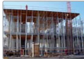
CONSTRUCTION Formwork and scaffolding
