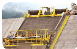
SLIPFORM CONCRETE PAVER FOR DAMS
